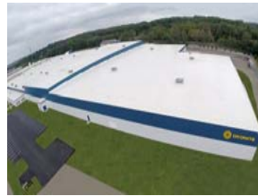
Cumberland, RI - Manufacturing Plant
