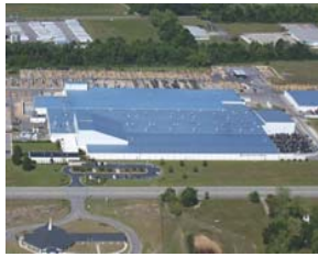
Orangeburg, SC - Manufacturing Plant
